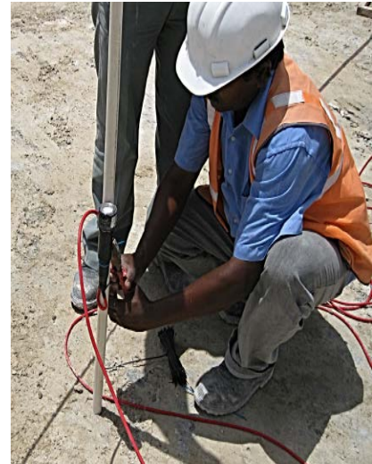
Figure 4.2 – installation by fully groutable method
