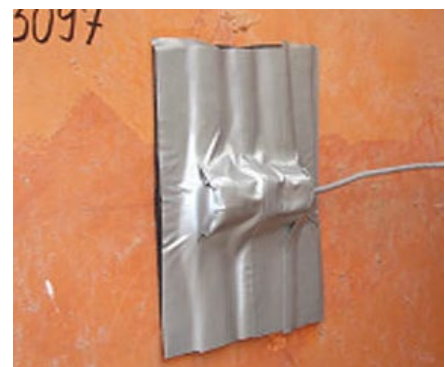
Figure 3.3 Further thermal protection by duct tape
