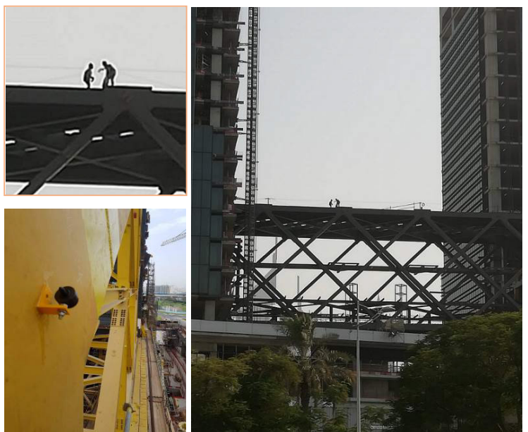
Installation of the prism targets on the Link Bridge
