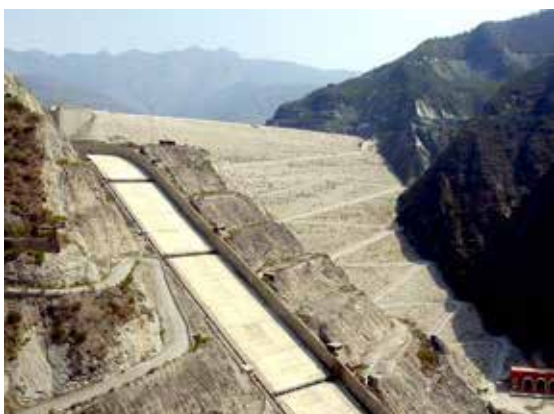
Tehri earth and rockfill dam, India
