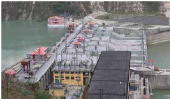
Teesta Concrete Gravity Dam, India
