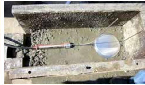
Concrete pressure cell being installed in Ghatgar Dam, India
