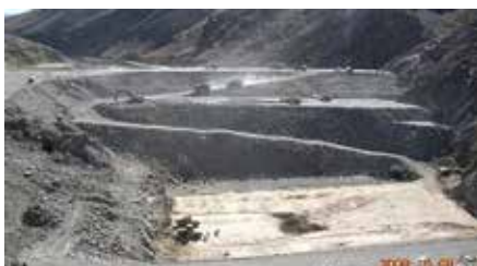
Work in progress at Salma Dam, Afghanistan
