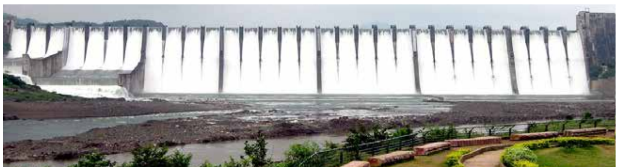
Sardar Sarovar Concrete Gravity Dam, India
