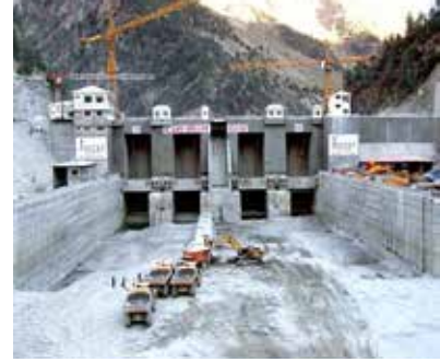
Karchham Concrete Dam, India
