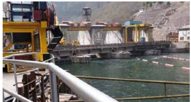
Chukha Concrete Gravity Dam, Bhutan
