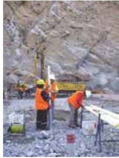
INCLINOMETER BEING INSTALLED IN EL PLATANAL ROCKFILL DAM, PERU
