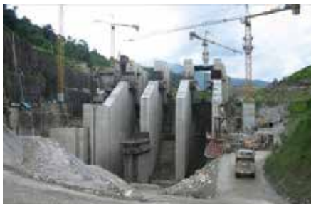
Work in progress at Middle Marsyangdi Dam, Nepal
