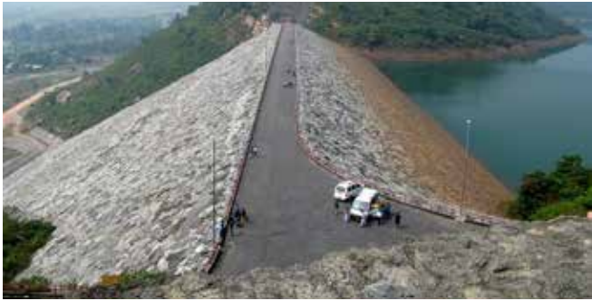
PURULIA EARTH DAM, INDIA
