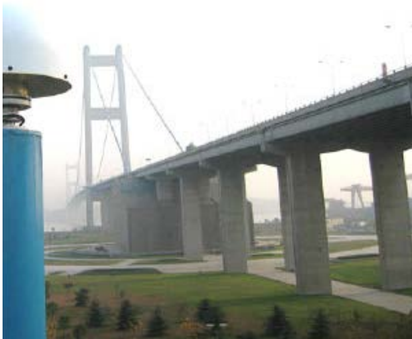
Reference GNSS station of a bridge monitored using GNSS rover stations
