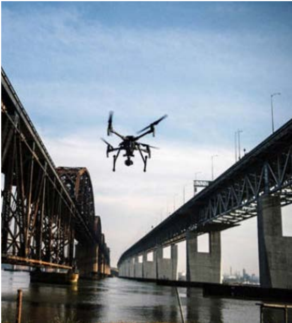
Bridge inspection using drone
